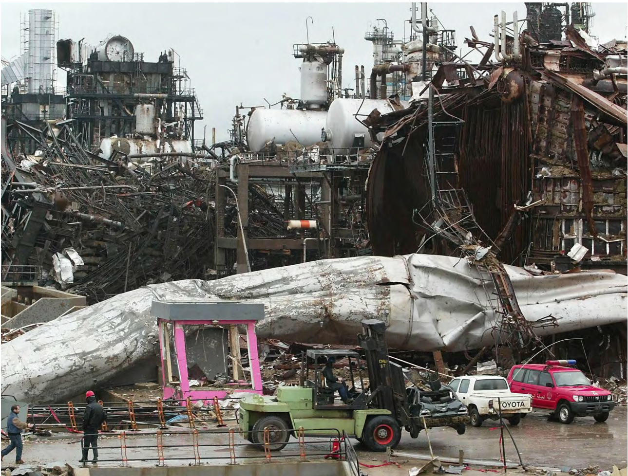
Skikda, Algeria – The LNG plant in Skikda stands in ruins following a devastating explosion on January 19, 2004. The blast, Algeria’s worst industrial disaster since independence, claimed at least 27 lives, injured many others, and severely impacted the nation’s gas-dependent economy.
